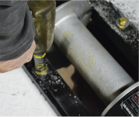
**4.** After successfully placing the winch on your truck, mount the frame. Using a total of eight grade 8, or "G8" bolts at least 3/8" thick is required. Lock washers as well.
