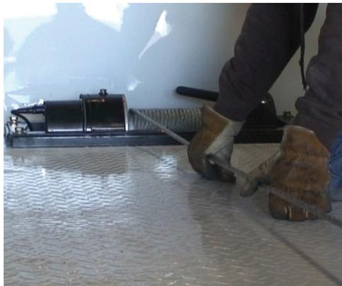
**6.** After connecting the cutoff switch and the ground line to the truck battery, install the wire rope onto the drum as shown. Feed the remaining length onto the winch drum while keeping the tension high.
